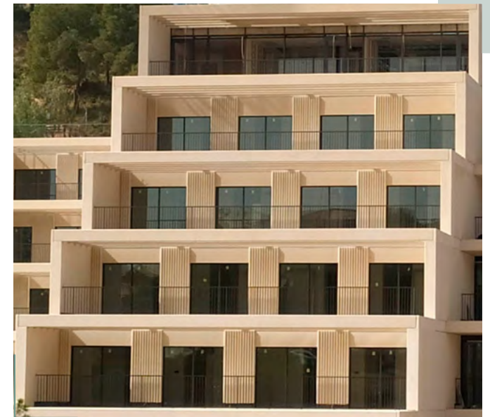
■ Residential with prefabricated structures in Malaga (Spain)
