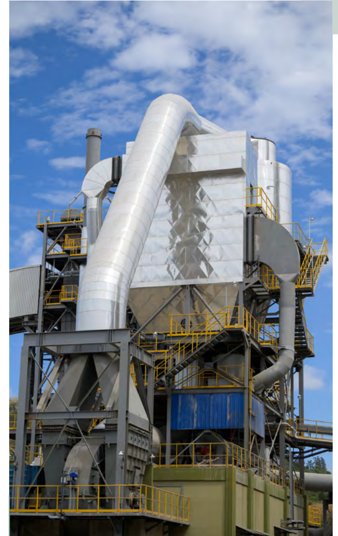
■ New vertical cement mil at Minas factory (Uruguay)
