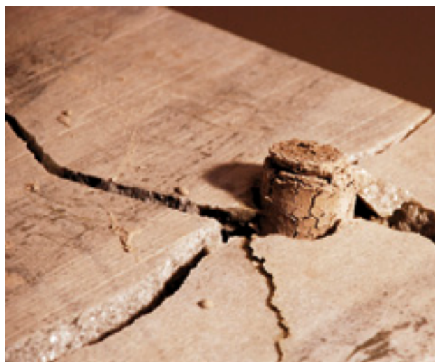
> Detail of application of "Betonamit" expansive mortar, Propamsa product, Spain
