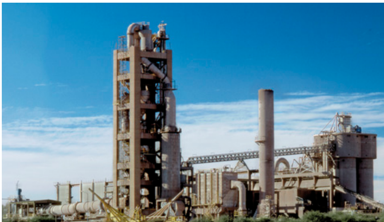
> San Luis plant, Argentina
