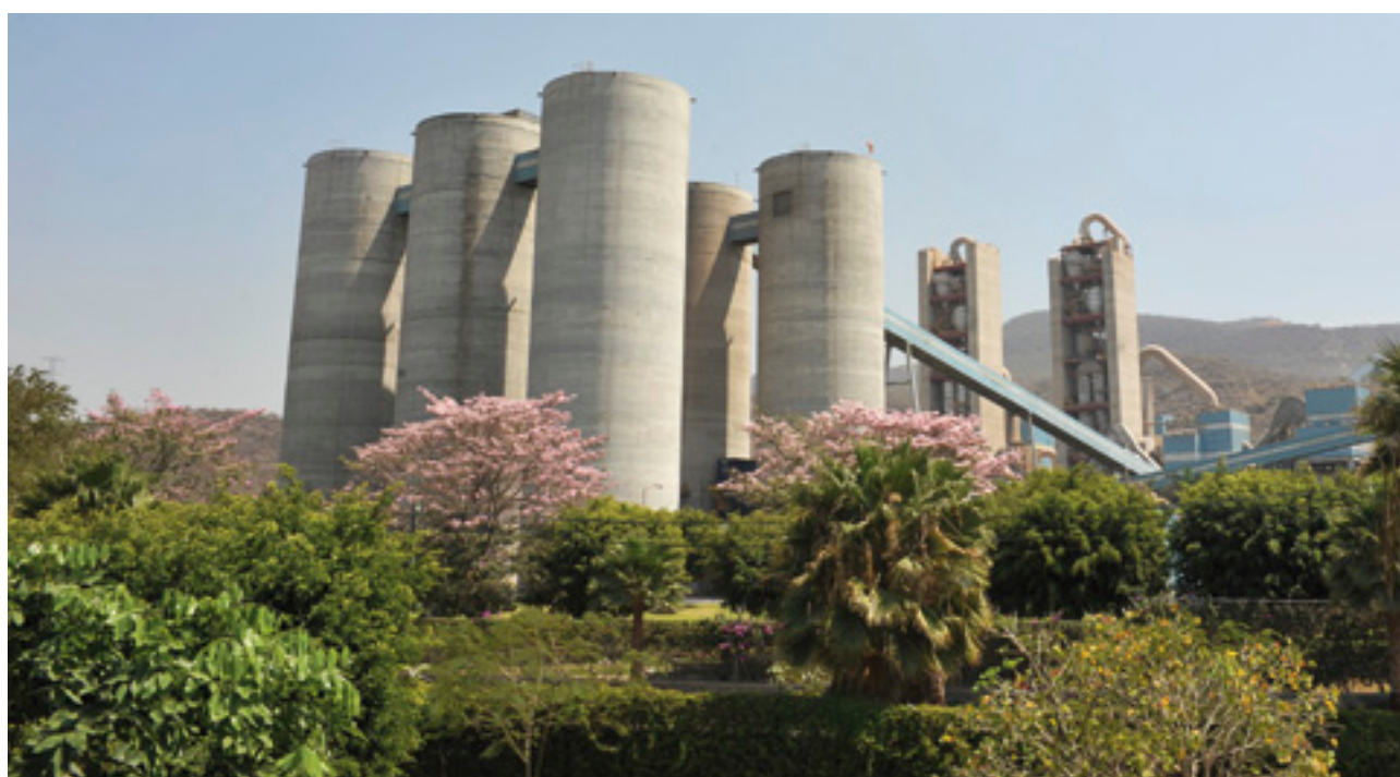
> Tepetzingo plant, Mexico
