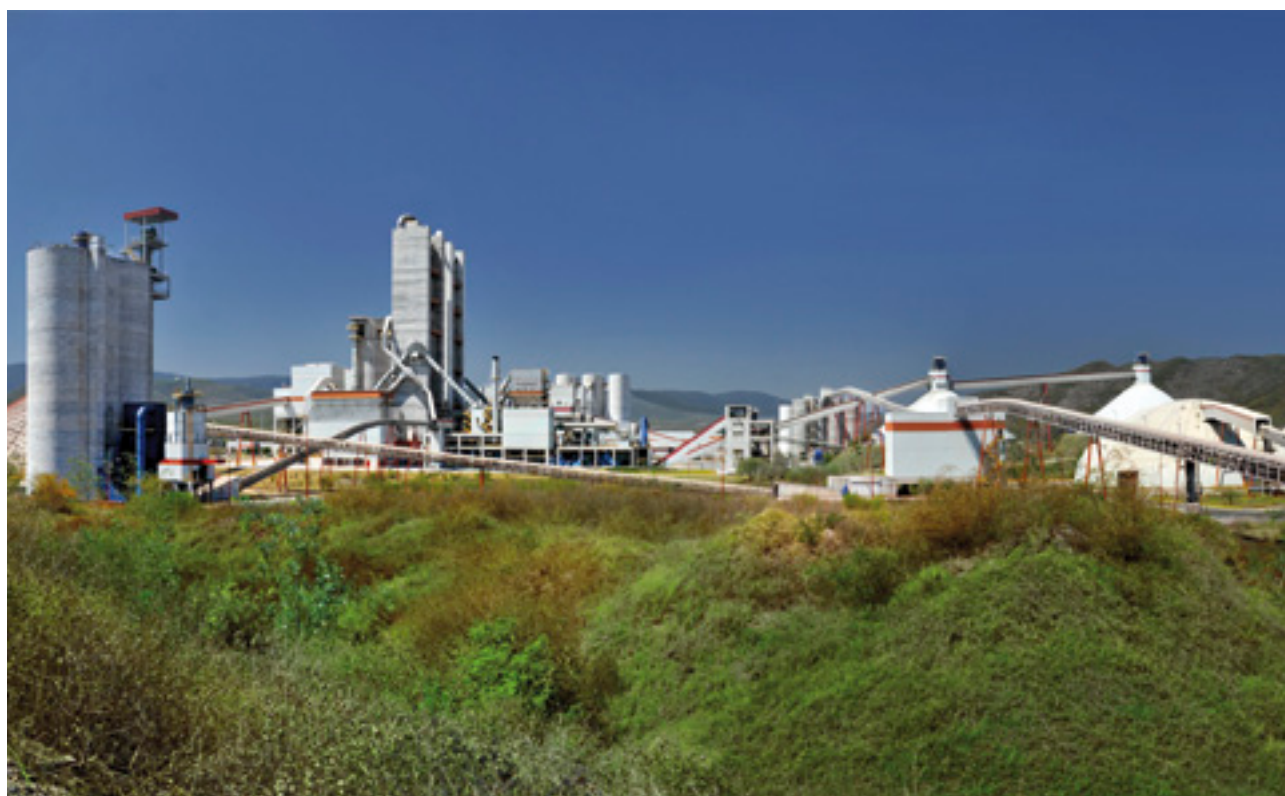
> Cerritos plant, Mexico
