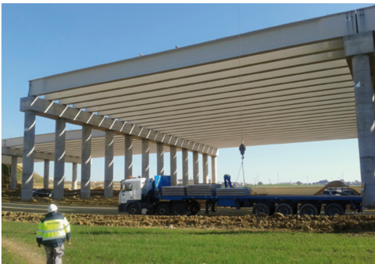
> Installation of a prefabricated structure, Precon, Spain
