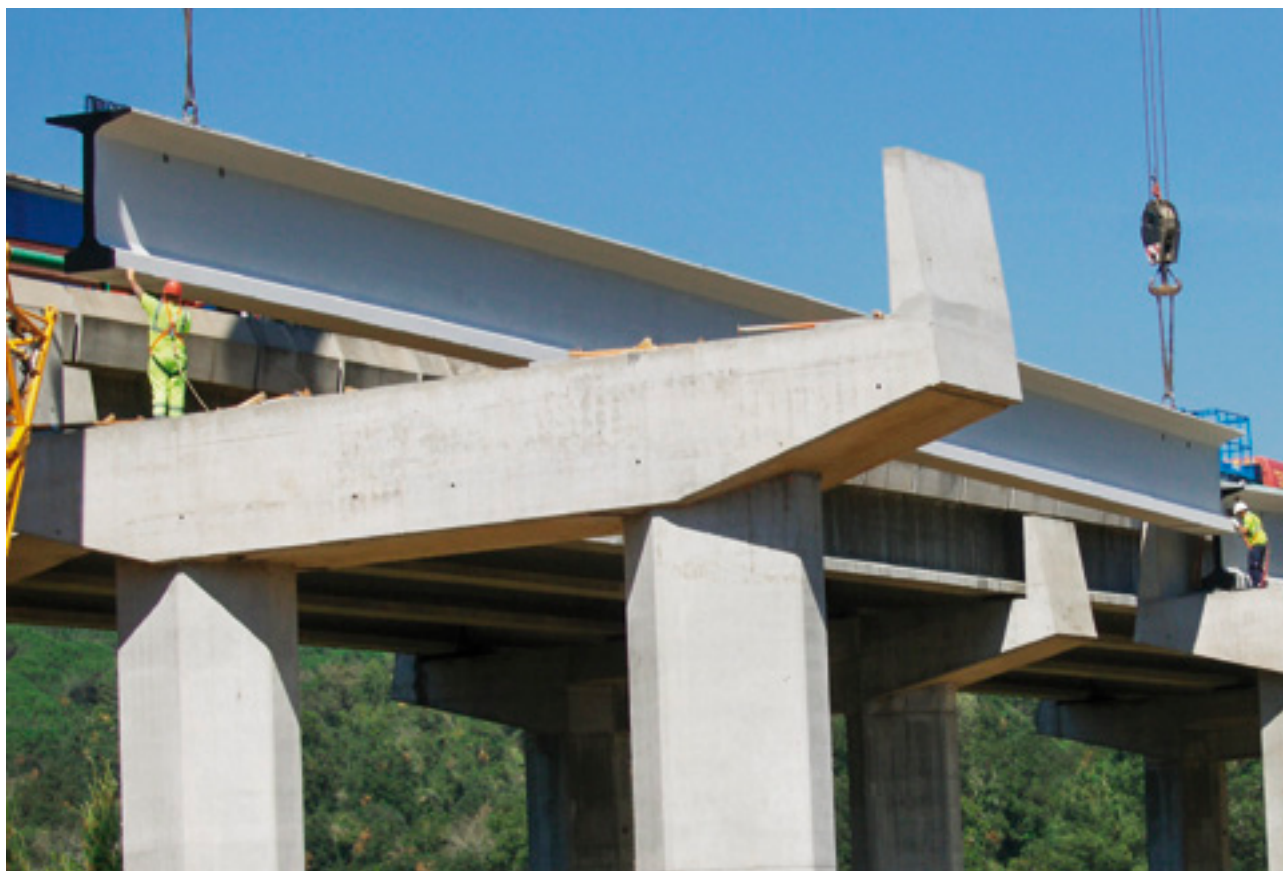
> Installation of a prefabricated structure, Precon, Spain
