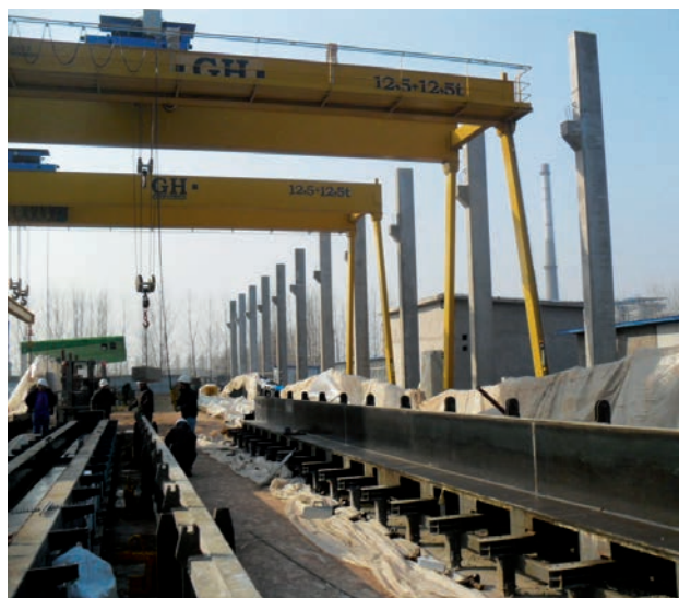
> Building work at the new factory of Precon in China
