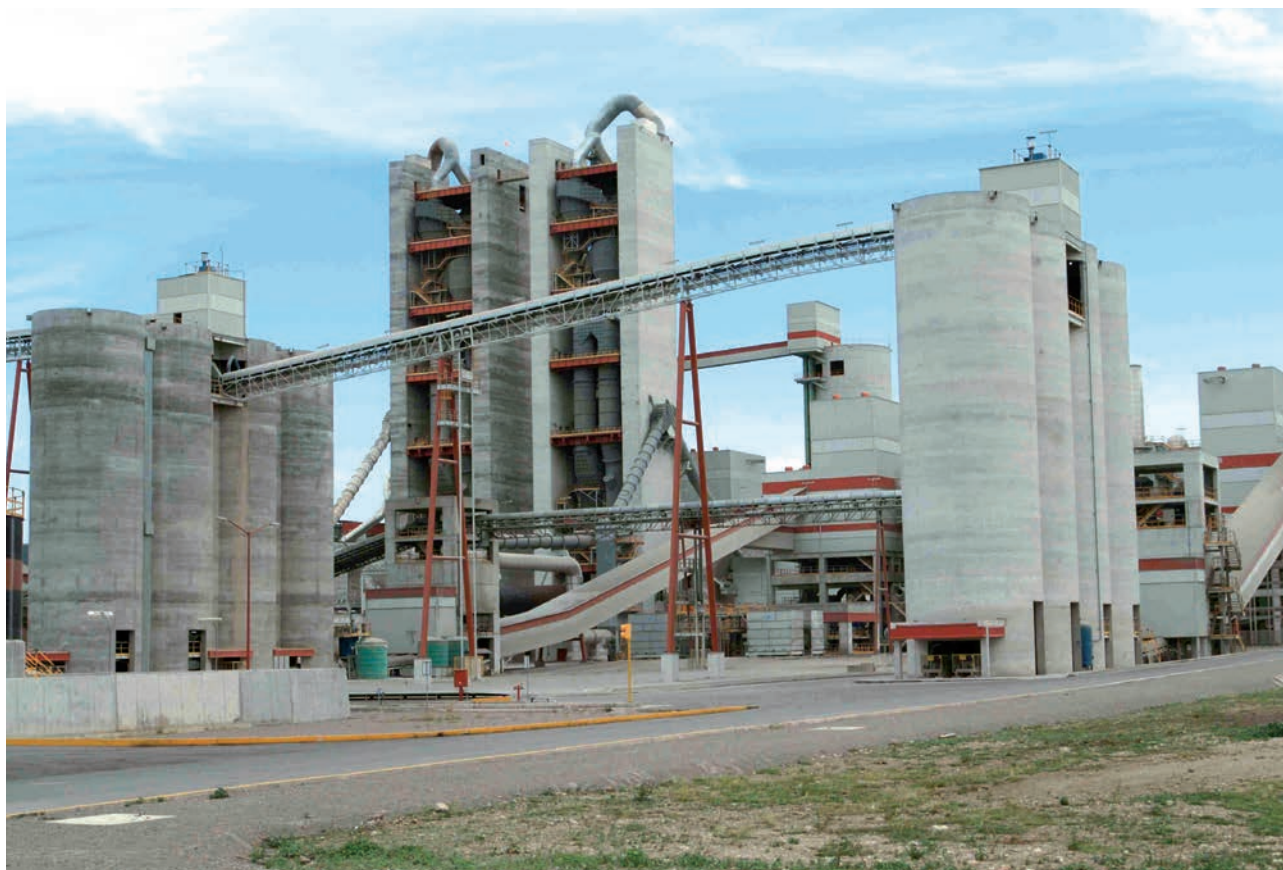
> Cerritos plant, Mexico
