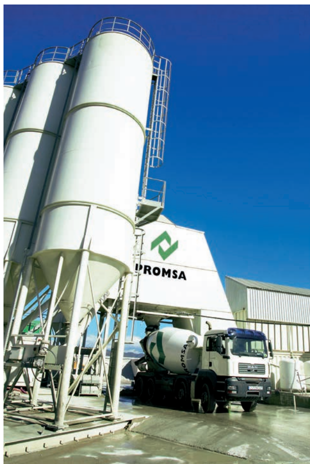
> Concrete production facilities, Promsa
