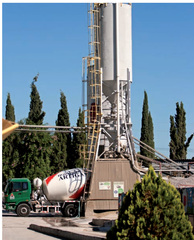
> Concrete production facilities, Cementos Artigas, Uruguay
