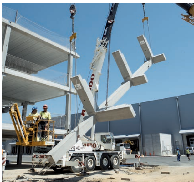
> Installation of a prefabricated structure, Precon
