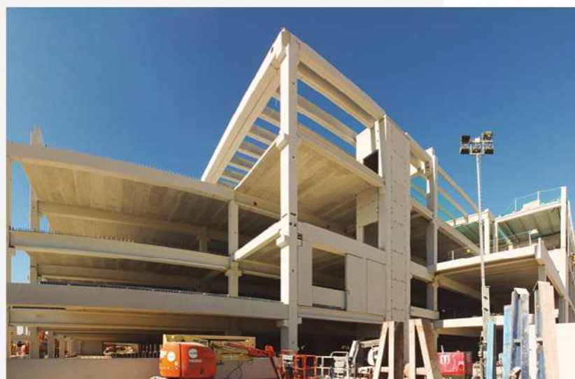
➤ Prefabricated structure of big surface. Precon.
