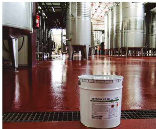
► Floor covering Epoxi. Betopox 92AR. Propamsa, Spain.
