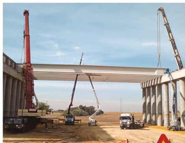
► Assembly of structures double T. Precon, Spain.
