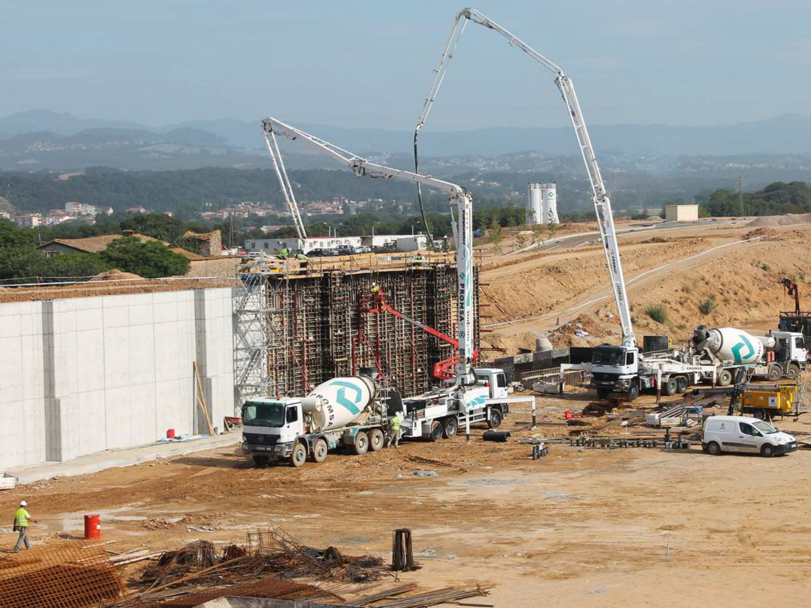
► Concrete supply, Pomsa, Spain.
