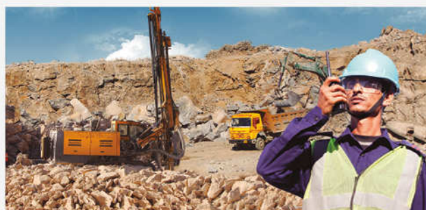
> Meghalaya's quarry facilities. India.
