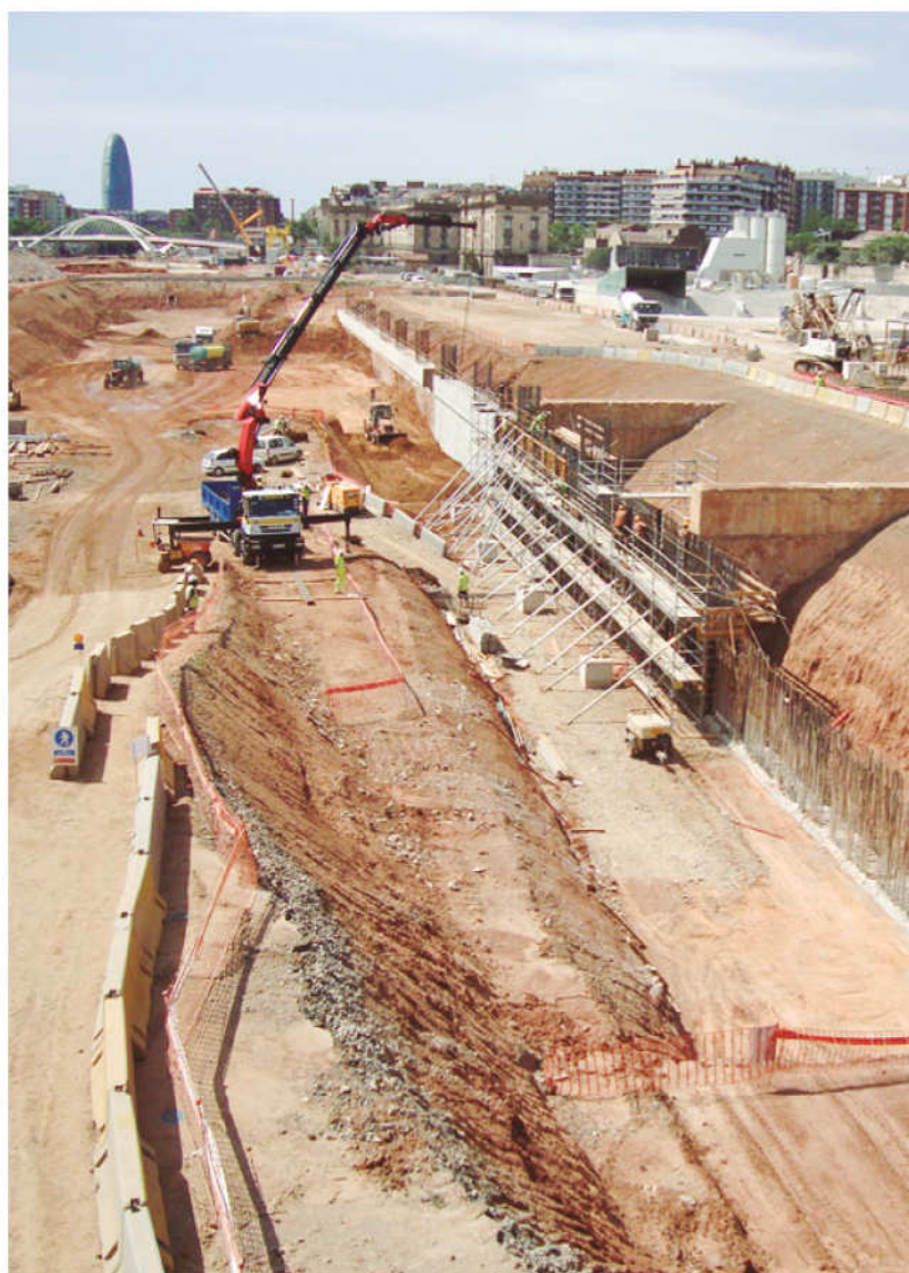
► Supply of concrete. La Sagrera Station. Promsa. Spain.
