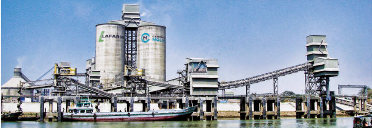
View of the pier factory Chhatak, Surma Cement.
