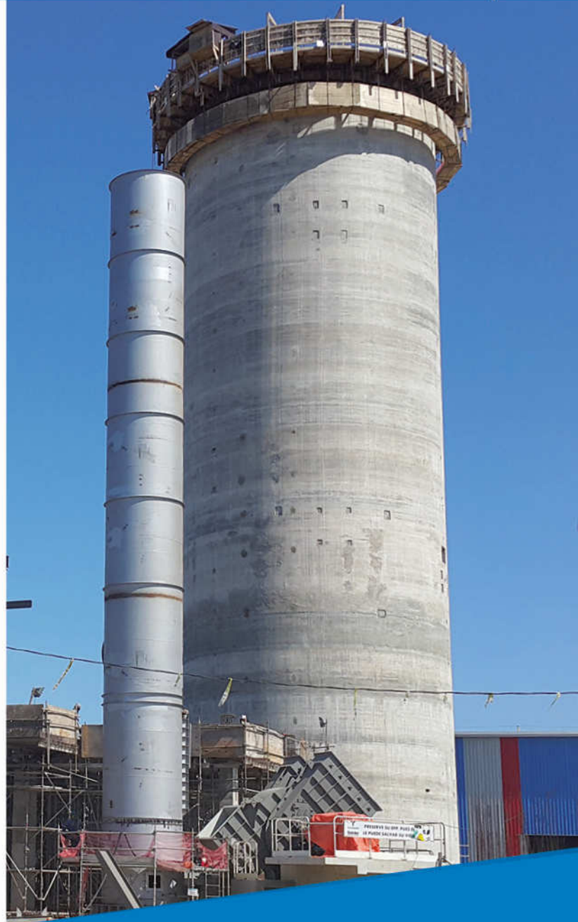
Construction of a cement silo for the new factory of Yacuses.
